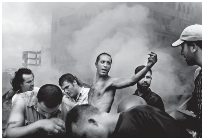
© Paolo Pellegrin/Magnum Photos, Civilians dig through debris for survivors just moments after an Israeli air strike destroyed several buildings in Beirut, Lebanon. 2006. (Bild: zVg IG Halle)
